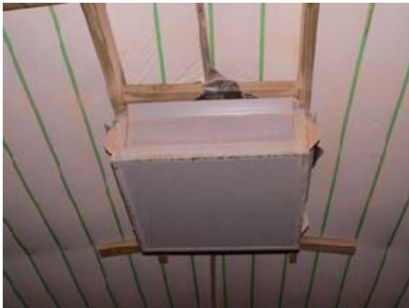
Attic inlet in the ceiling of a broiler house
