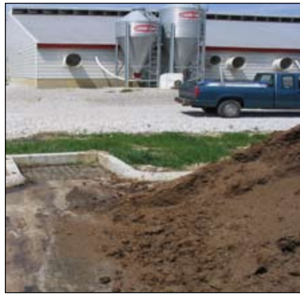
Figure 8. Mortality composting leachate entering drain to travel to existing lagoon.
