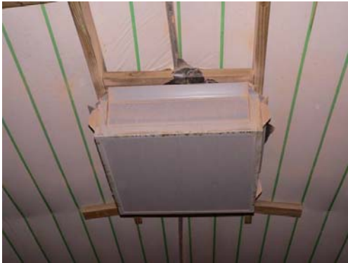
Figure 1.25 – Photograph of an attic inlet
