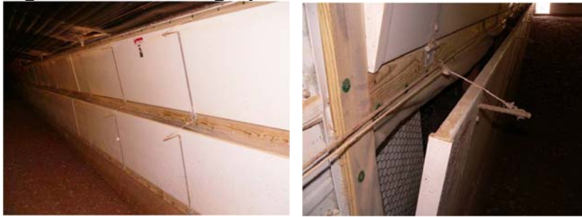
Figure 1.20 – Photograph of tunnel doors
