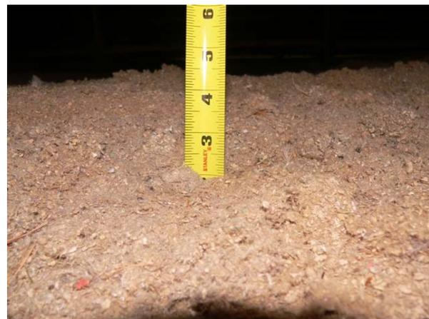
*It is usually cost effective to add 3-5 more inches of insulation to ceilings when the existing insulation is less than 3 inches thick.*
