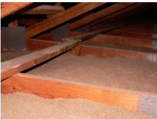
Insulation in the attic of a broiler barn
