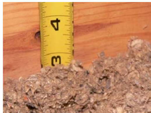
Measuring insulation in attic
