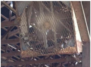
4. **Fans are placed too far apart across a row of fans**. In Picture 4, additional fans could be added to eliminate the dead space between fans. These types of fans are generally designed to blow forward, not necessarily to the side. During hotter temperatures, cows may be found lying in rows directly in front of the fans, showing that they prefer the areas with more airflow.
