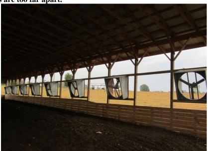
5. **Not enough fans over freestalls (Picture 5).** A row of fans should be present for each row of freestalls. In the picture below, only one row of fans is in place. Adding a second row of fans would increase air flow to the cows resting in the freestalls.
