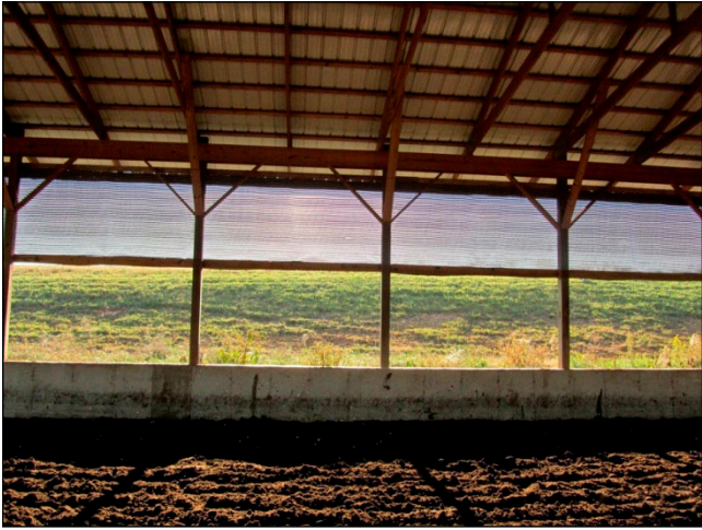
Figure 31. Shade cloth may help with cow distribution, particularly in barns with a north-south orientation. The shade should not block airflow.
