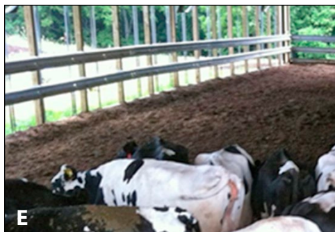
Figure 15. Barrier topper options include (A) steel cable, (B) pipe, (C) fence panel, (D) wood planking, and (E) highway guard rail.
