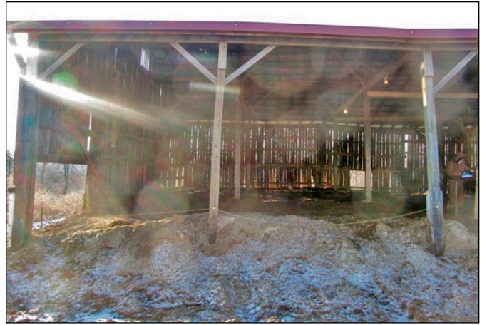
Figure 27. This barn is too closed in to allow for compost drying and air removal.
