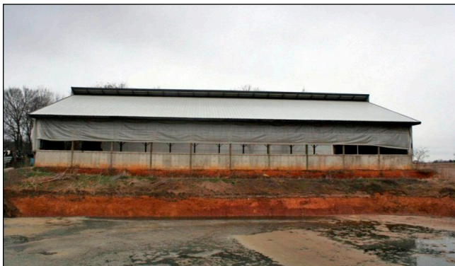
Figure 30. Cold winds blowing across the pack quickly remove the heat needed for composting. Thus, curtains are recommended in the winter. Curtains should be placed at least on the side with predominant winds.
