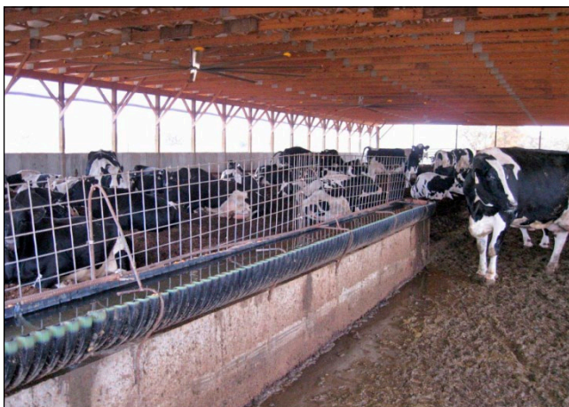
Figure 24. This barn incorporated a drainage pipe with free-flowing water along the entire length and opposite of the feed alley.
