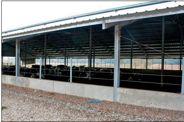
Figure 26. High, open sidewalls maximize cross ventilation. A minimum 12 foot opening should remain between the top of the retaining wall and the bottom of the barn eave.
