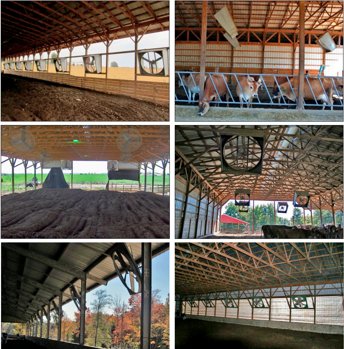
Figure 41. Properly positioned fans help cool cows and dry bedding material. They should be placed to supplement, not fight, natural airflow. Follow manufacturer recommendations for spacing and placement.
