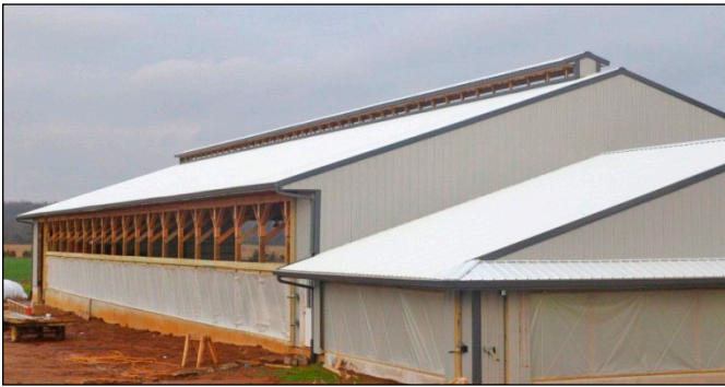
Figure 34. This uniquely designed barn takes advantage of the most important principles for ventilation. However, the completely enclosed end attached to the milking parlor may limit airflow, and the overhangs are too short.
