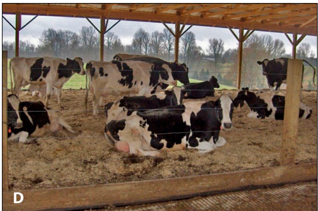
Figure 13. Because the pack area serves a dual purpose of providing resting space for cows and storing manure, many producers build a retaining wall around the pack with either (A) cast-in-place concrete, (B) wood plank, or (C) highway guardrail. Other barns (D) have minimal to no separation between the pack area and the outside of the barn or feed alley. All designs can work well.
