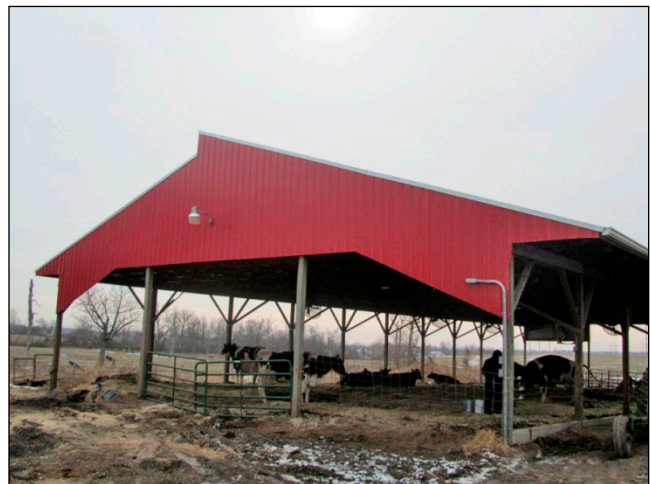
Figure 36. These designs share all the features of the first design except for the open ridge. These use an overshoot roof with an opening large enough to allow air removal from the top of the barn. The disadvantage to these is that when the wind blows toward the opening, it may actually push hot or stale air back into the barn in warmer months and cold air in the winter.
