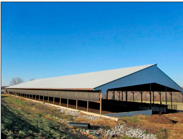
Figure 36. These designs share all the features of the first design except for the open ridge. These use an overshoot roof with an opening large enough to allow air removal from the top of the barn. The disadvantage to these is that when the wind blows toward the opening, it may actually push hot or stale air back into the barn in warmer months and cold air in the winter.
