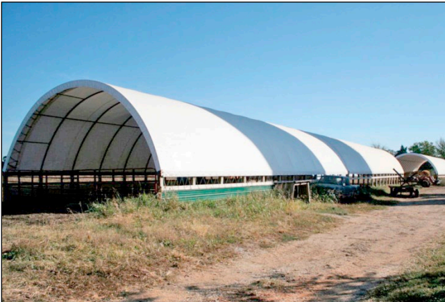
Figure 10. A few producers have used hoop structures for compost barn housing.
