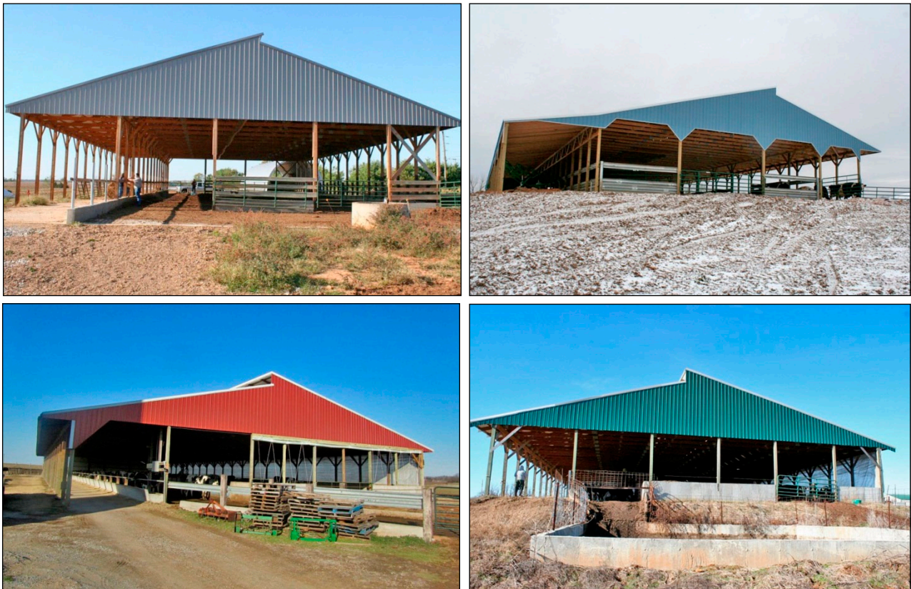
Figure 39. When the opening of the overshoot ridge is too narrow, the design restricts air removal from the top of the barn and is not generally recommend.
