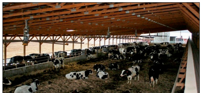
Figure 61. This barn incorporated a concrete barrier to separate the barn into two management groups. Additionally, a catwalk was added to the barn for cow observation.
